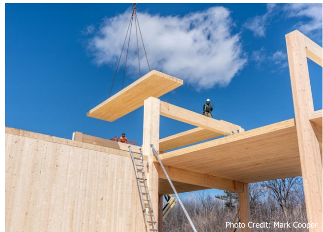
Installation of mass timber elements on the 2-storey structure.
